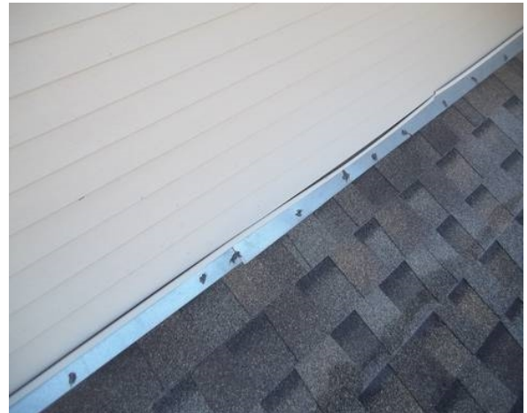
Secure siding as required to reduce further damages.
