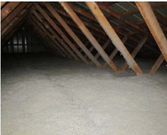
Garage attic, apx. 4 inches of blow in insulation.
